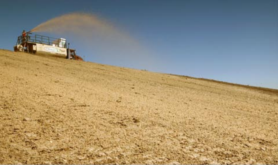
GeoPerm™ applied on 2:1 Slopes
