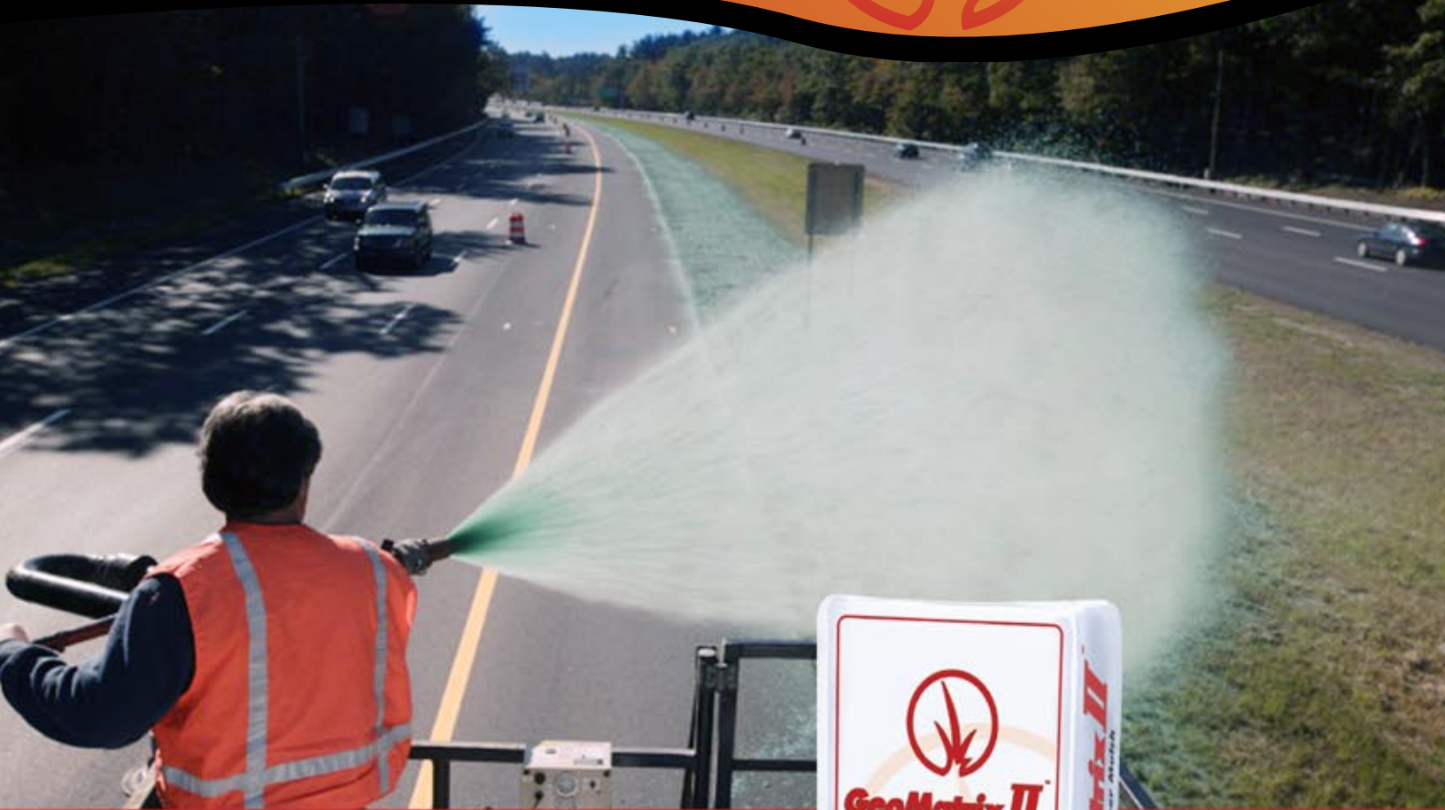
GeoMatrix II being applied from tower
